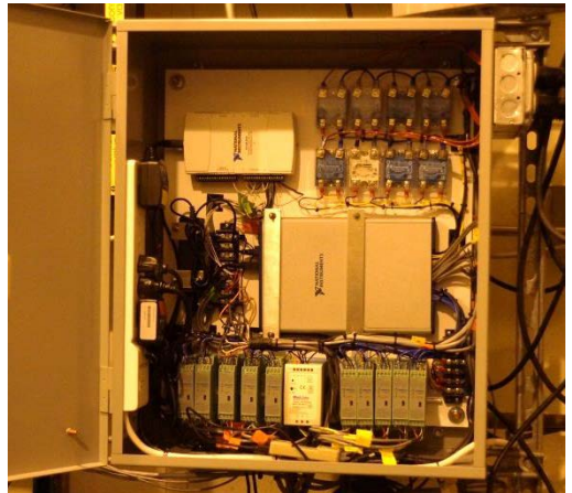
Data acquisition and control hardware interface
